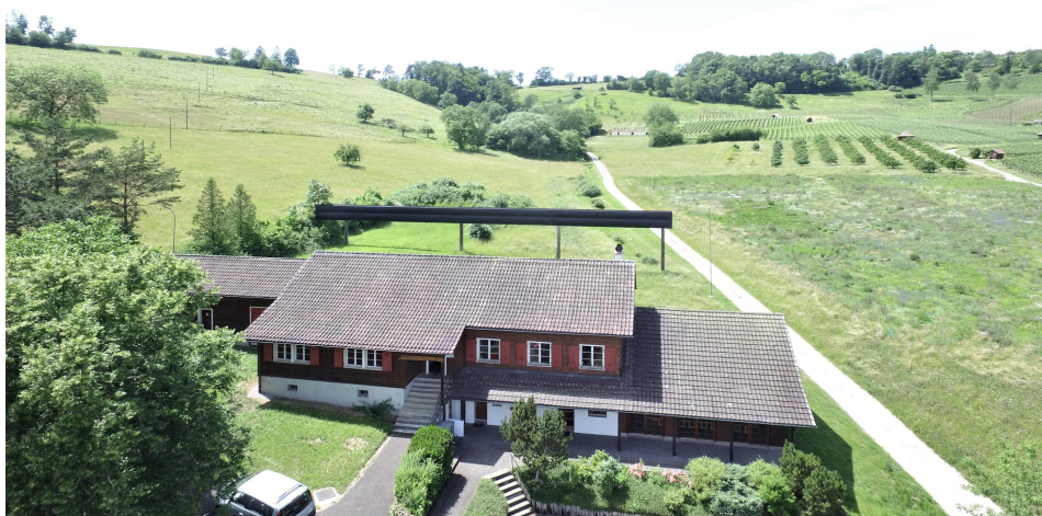
Schiessanlage "Waatile" in Hallau SH
